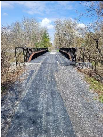
Bridge recently rehabilitated with guard rails and rubber mats to improve crossing conditions for pedestrian/equestrian/dog walking users.
