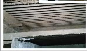
Sludge and calcium buildup in a condenser
